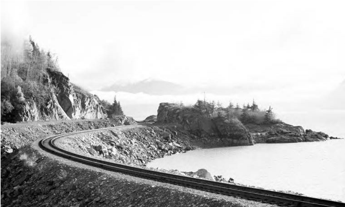
Figure 1. View of Beluga Point over railroad tracks, looking southeast, 1939–1959.
