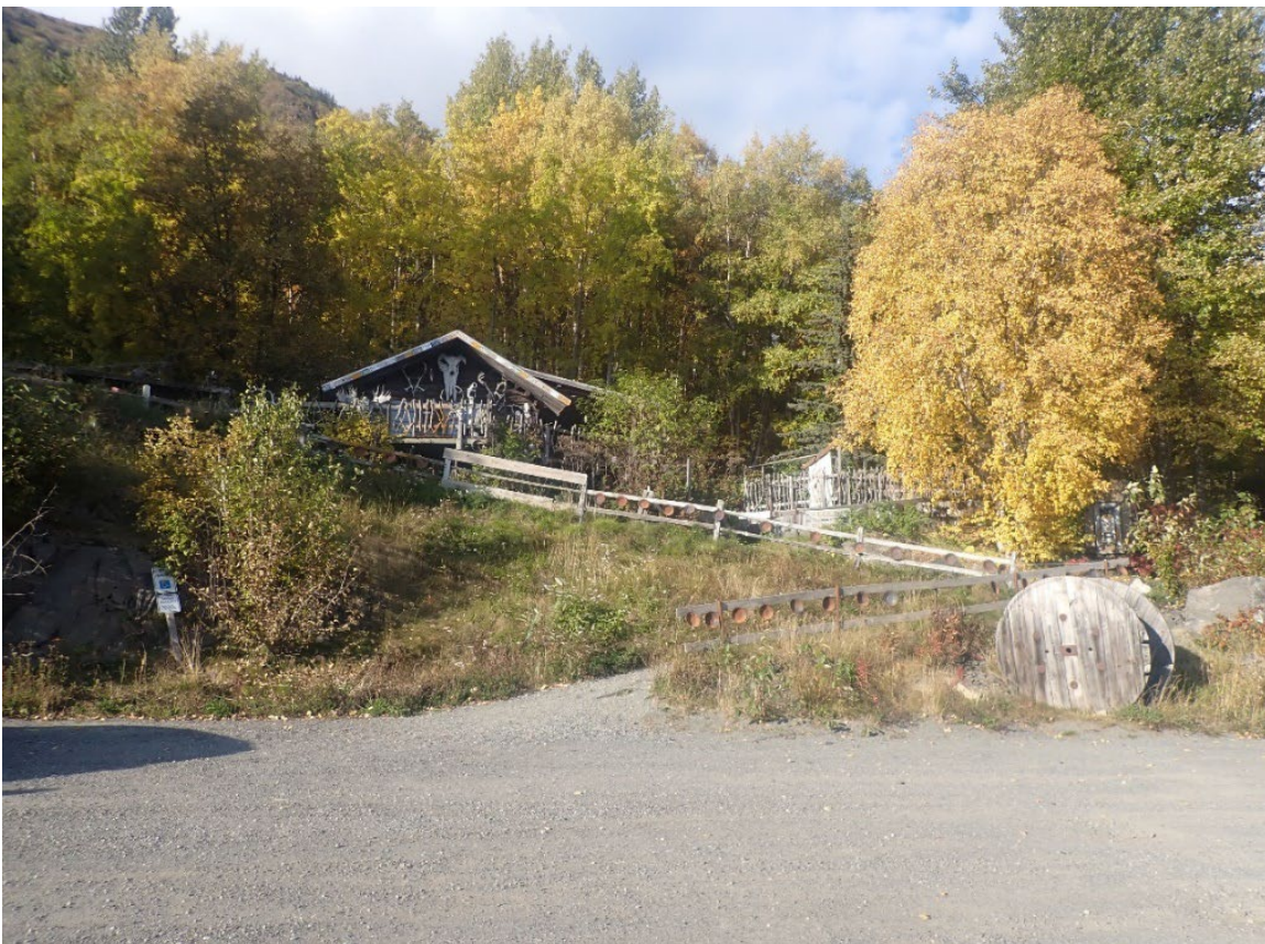
Figure 6. SEW-00412 (Indian Valley Mine), view north, log cabin at center and the assay office's roof at left.
