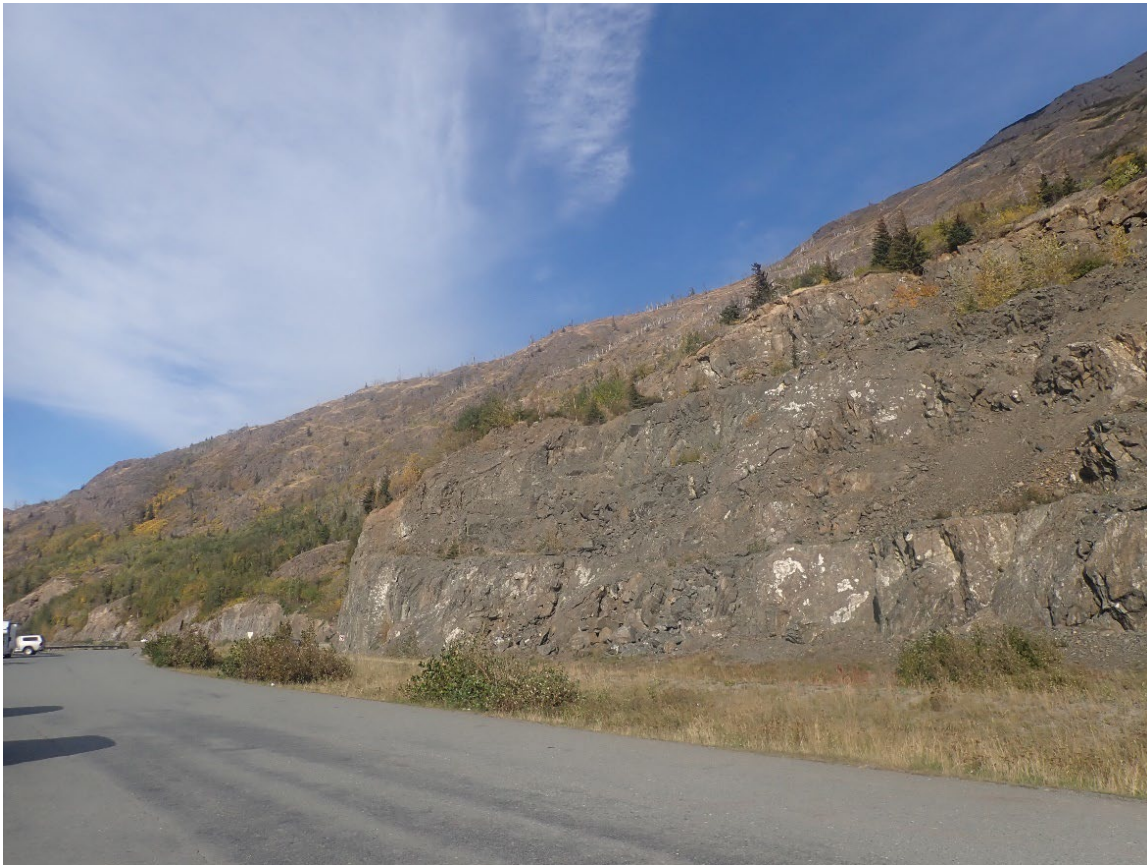
Figure 2. Steep rock face opposite the Beluga Point wayside, view northwest.
