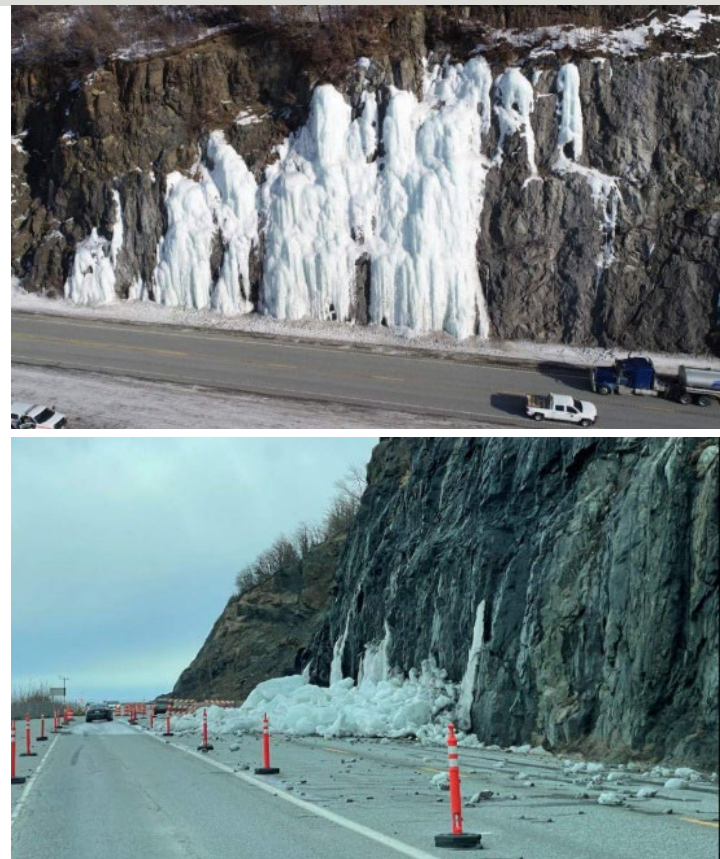
Figure 2-3. Ice buildup at Seward Highway MP 113.2 (winter 2020; top) and ice collapse at MP 113.2 (March 2022; bottom).
