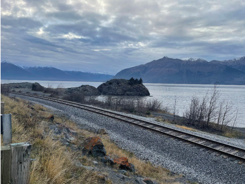
Photo 23: Looking southeast at the Beluga Point from a scenic overlook located at Mile 110 of the XSC. (November 2, 2023)
