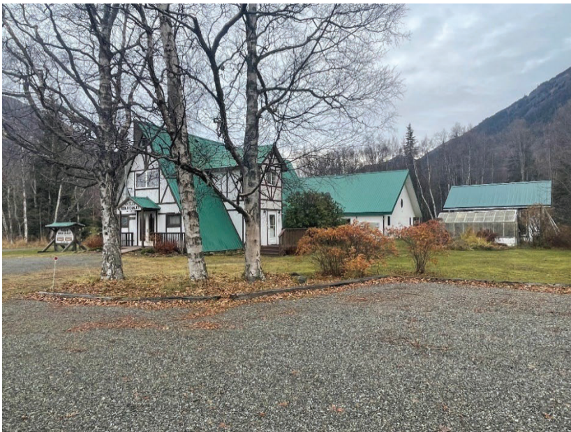
Photo 12: Looking northwest at the Valley Bible Chalet and associated structures, located near Mile 103 of the XSC. (November 2, 2023)
