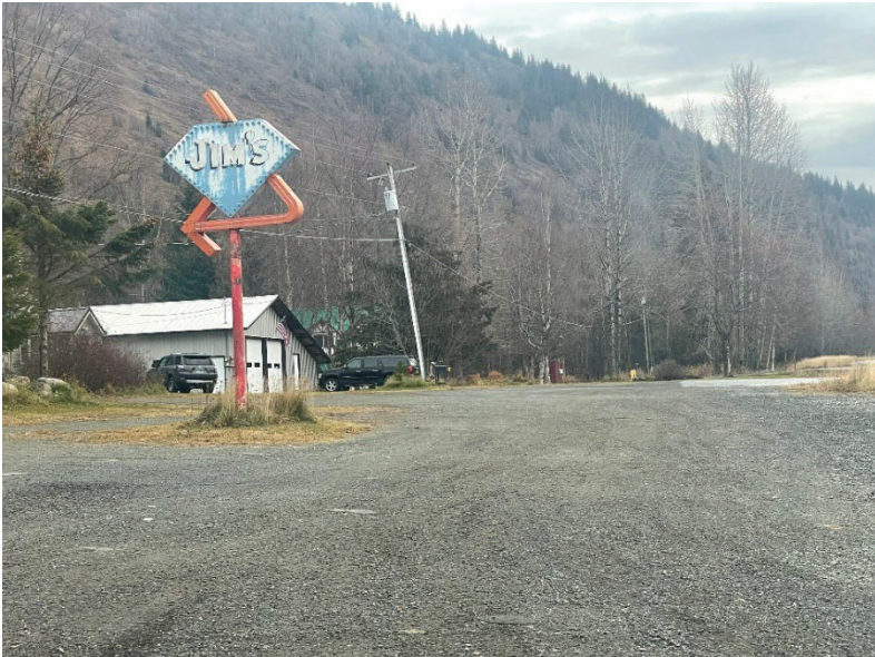
Photo 14: Looking south at Dimond Jim's Liquor & Gift shop, unpaved parking lot, residential structures, powerlines, and pole-mounted transformer located near Mile 103 of the XSC. (November 2, 2023)
