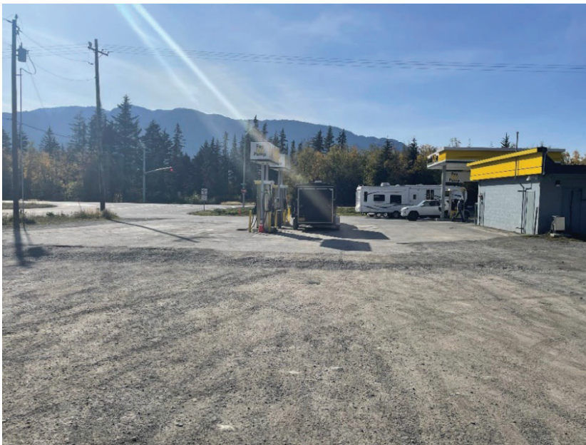
Photo 8: Looking southwest at pump islands and the parking lot of 29383 Seward Highway. (September 27, 2023)
