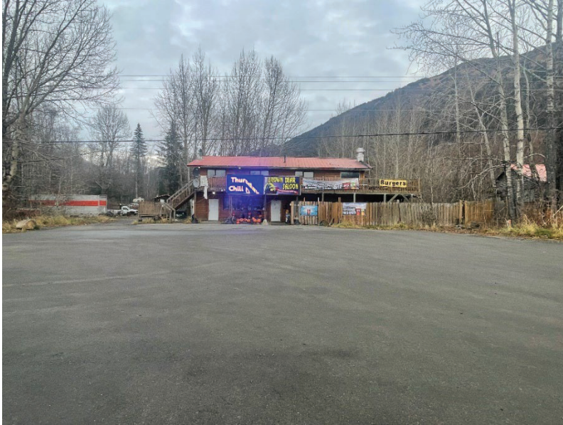
Photo 15: Looking west at the Brown Bear Saloon, located near Mile 103 of the XSC. Several 55-gallon drums, a boat, parked cars, and connex were observed near the structure. (November 2, 2023)
