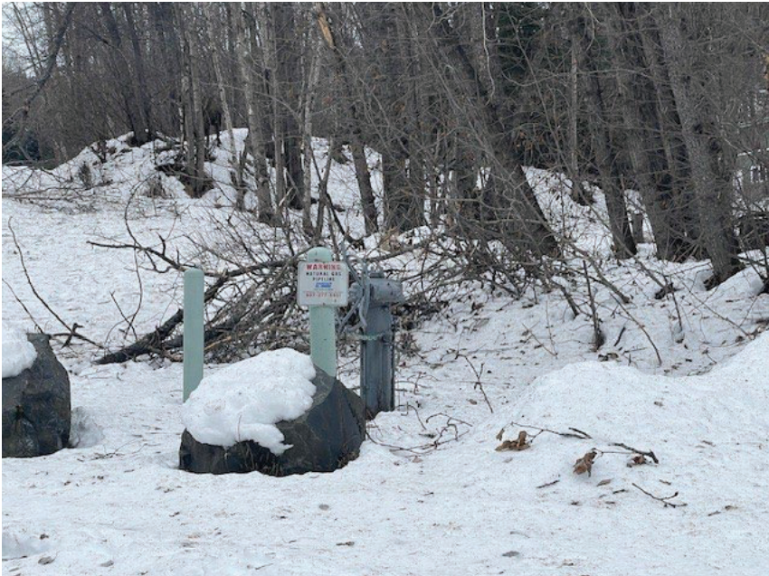
Photo 28: Looking northeast at a posted sign and access port for an ENSTAR natural gas pipeline located near Mile 115.25 of the XSC. (December 4, 2023)
