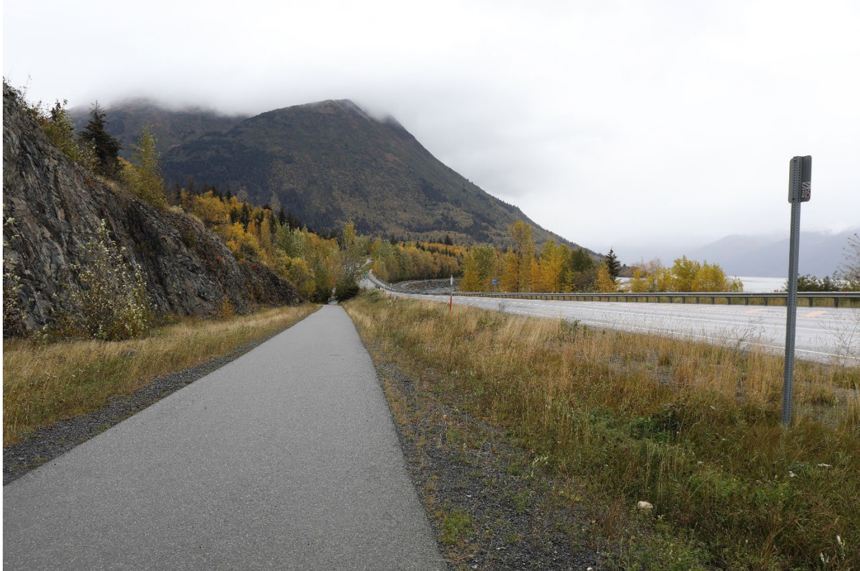
Figure 3-5. View from the Indian to Girdwood Bike Path before crossing Bird Creek.
