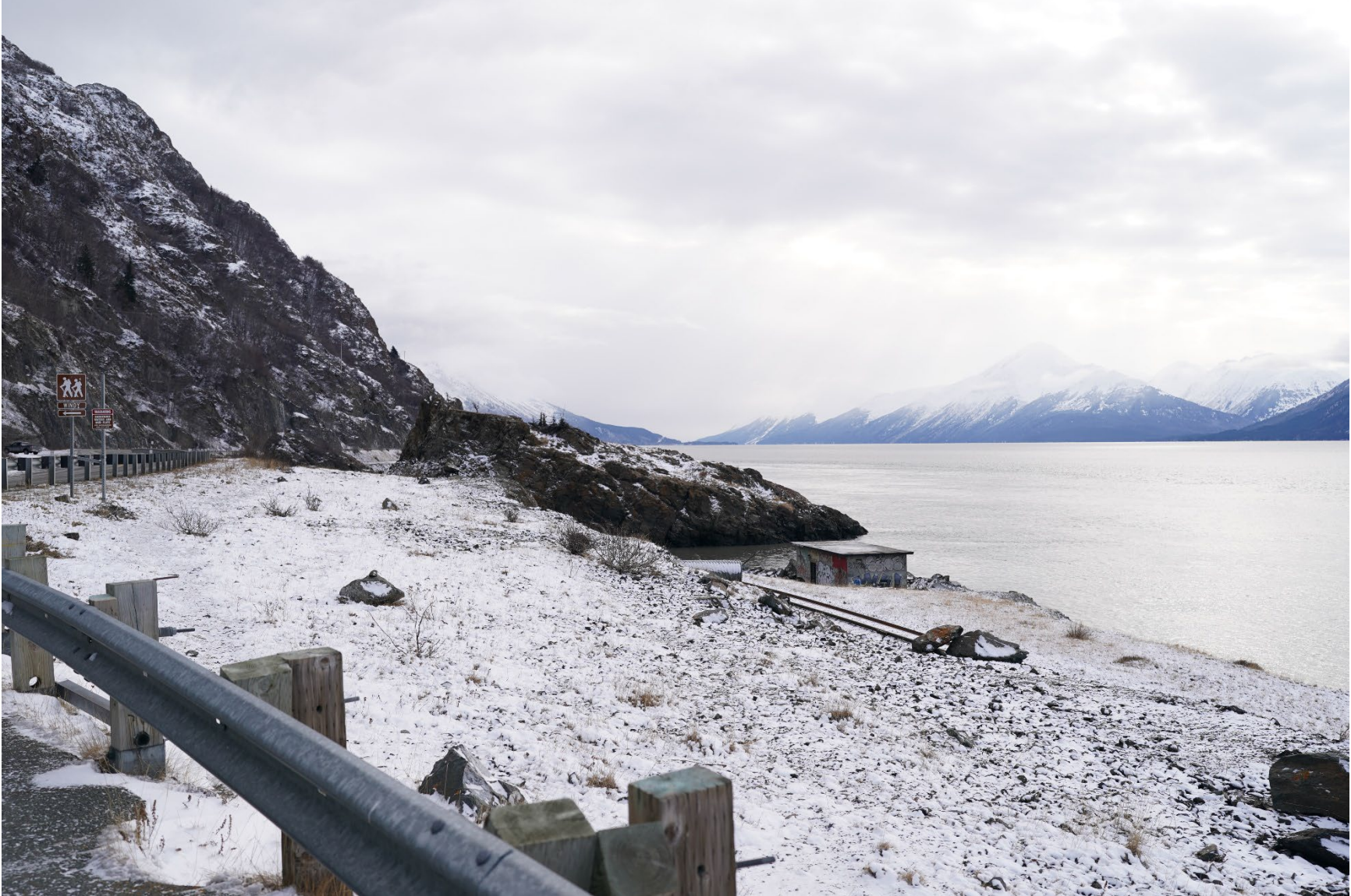
Figure A-9. Existing view of the Windy Scenic Overlook area, from MP 106.75, facing south.
