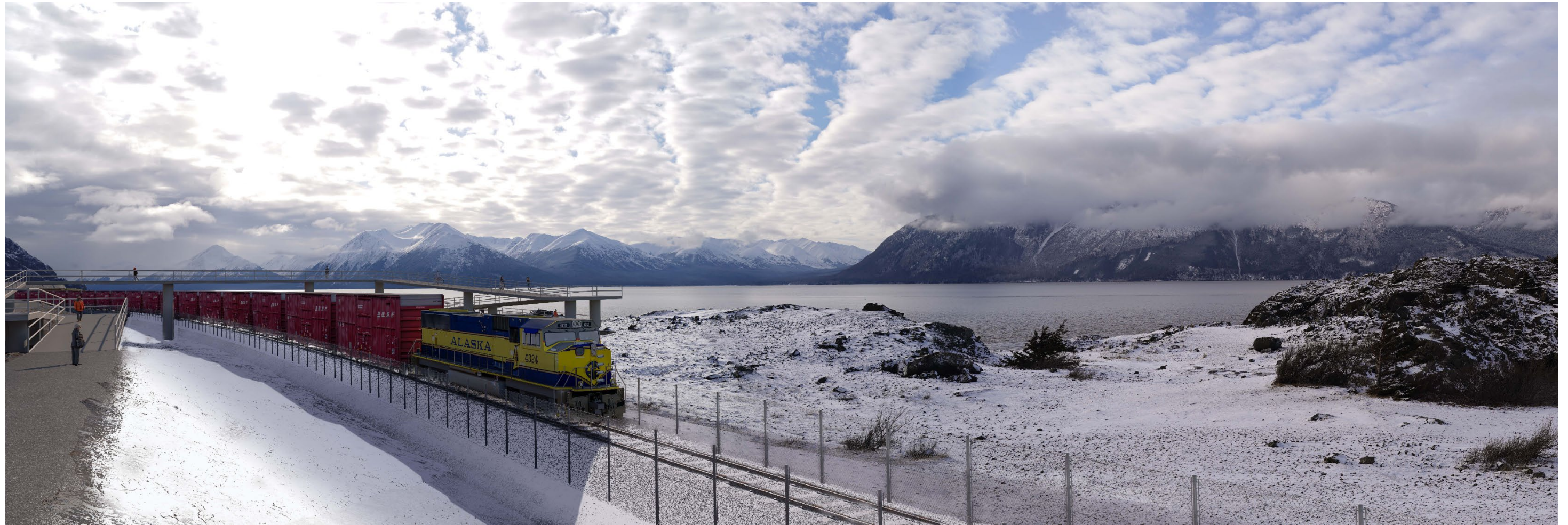
Figure A-8. Visual simulation of Beluga Point, from MP 110.25, facing south. Note that the rendering shows the ability of a double-stacked train to travel under the pedestrian overpass.
