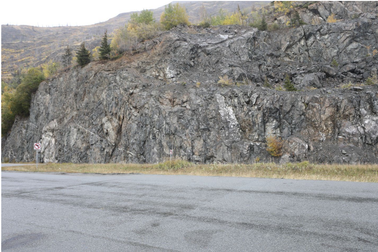
Figure 3-2. Example of previously blasted, weathered rock face.
