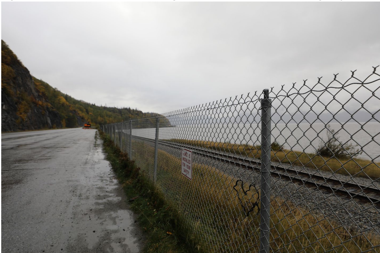
Figure 4-1. Example of a fence separating ARRC tracks from the Seward Highway.
