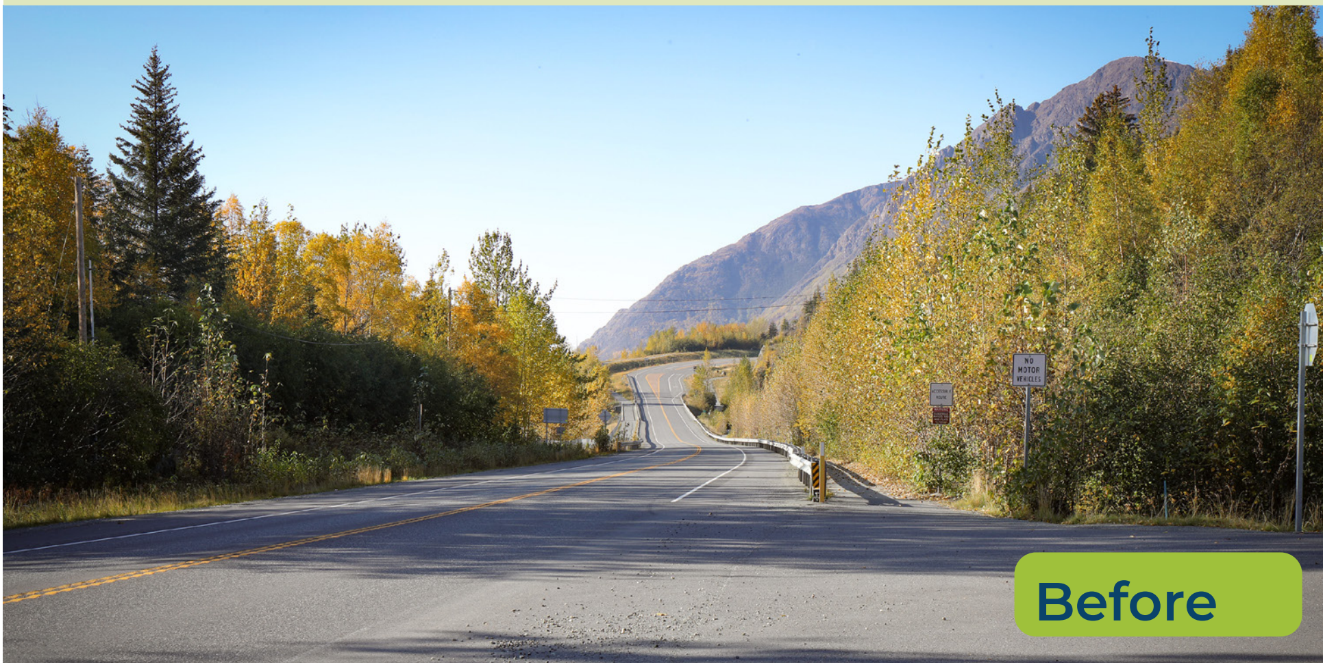
Bird Creek Looking North
